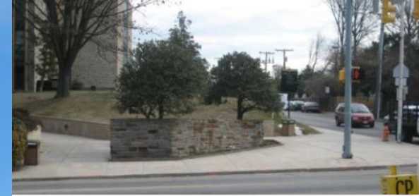
Before: Existing Conditions at Northeast Corner
