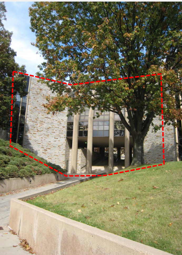
Existing Conditions: Diagonal walk leads under existing building which was demolished to accommodate new infill building. Diagonal walk provided access to the Academic Quad from Charles Street.
