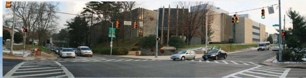
Before: Existing Conditions at Northeast Corner looking to Donnelly Hall
