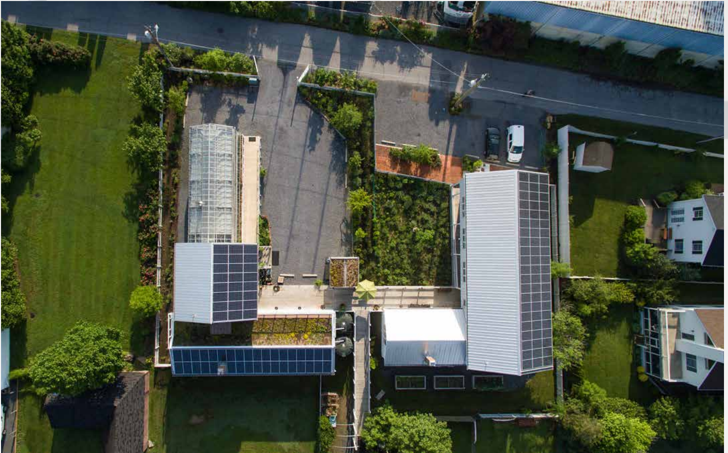
Aerial Project Scope Image
