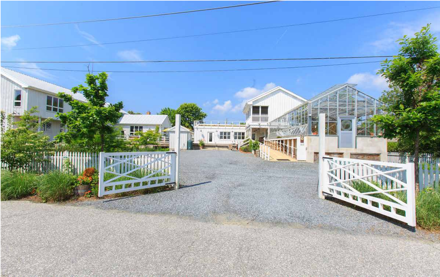
After 101 & 103 Mill Street Project
