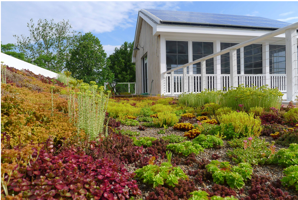
Installed Solar Panels & Green Roof
